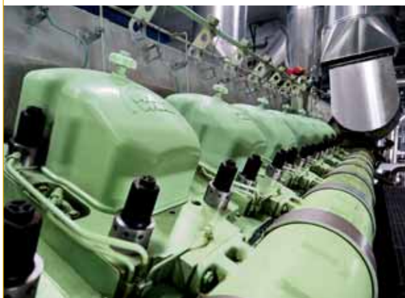
MAN engine DIESEL 18V 32/40
